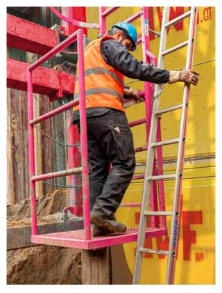
Depending on where the ladder is attached to the lower platform, a chain is detached on the right or left side using the carabiner fastening.
