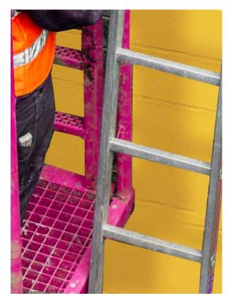
For the last section of the descent into the pit a lean-to ladder is used, which can be attached to either side of the lower shoring ladder platform.
