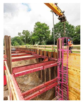
Putting the ladder in place using an excavator. Fall protection must be closed at the edge areas during installation.
