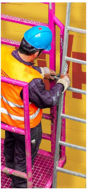
The ladder upright must be secured tightly to the side of the shoring ladder using a chain to prevent the ladder from tipping over to the side.
