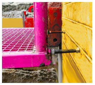
On the lower platform and ideally on every second extension piece of the shoring ladder there are two adjustment screws (SW30) for vertical alignment. The minimum distance between ladder and shoring surface must be 150 mm to ensure that feet can be placed securely on the rungs.
