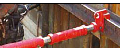
End hooks for steel walings special solution
